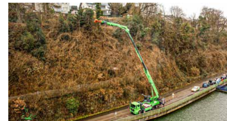
Working possible without blocking both lanes.
