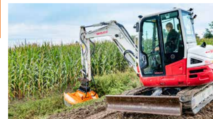
Mulcher at slope maintenance.
