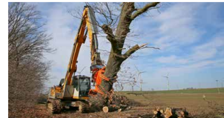
Maintenance work along traffic roads and routes.
