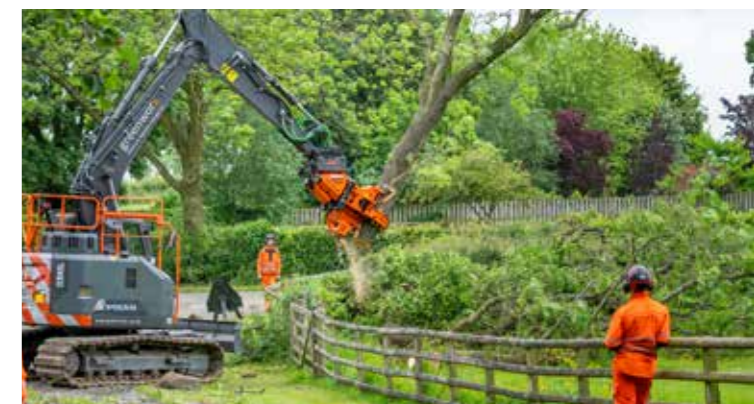
Maintenance work along traffic roads.
