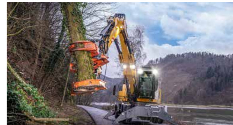
C350 during forest edge maintenance.
