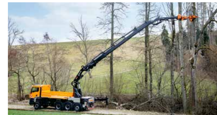
Working safely with high reach.
