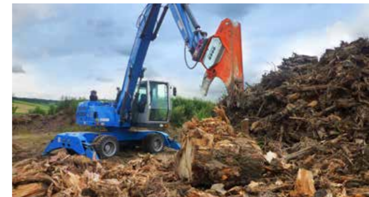
Used for clearing the soil.
